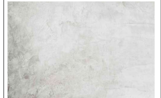
DIRTY/OFF-WHITE STUCCO FINISH
