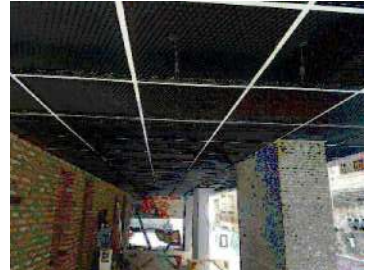
RCP-G METAL SCREENED CEILING
