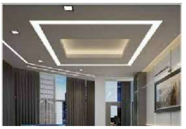
RCP-B COVE CEILING IN GYPSUM BOARD MATERIAL PAINTED IN FLAT WHITE LATEX PAINT
