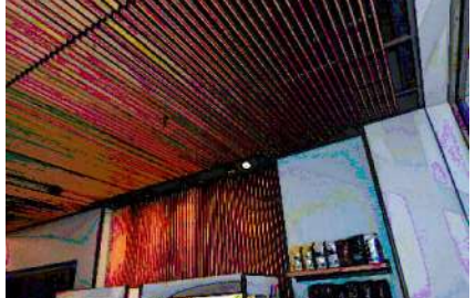
RCP-F WOOD STRIP/PLANKS CEILING
